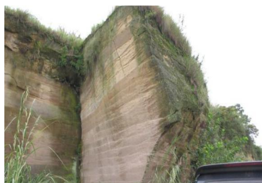
(b) Site of Dangerous Rock Mass
